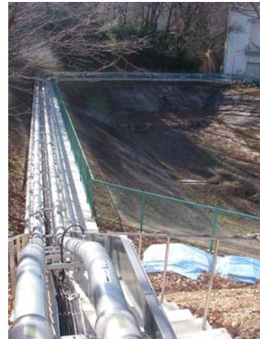
Fig. 2 Insulated double-tube (outside the laboratory building)
