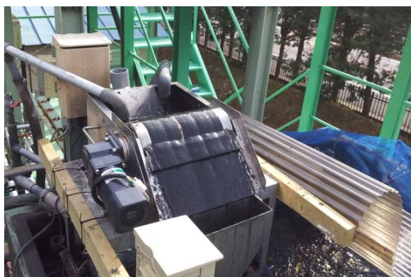
Fig. 1 Drum-type magnetic separation system installed at pilot plant
