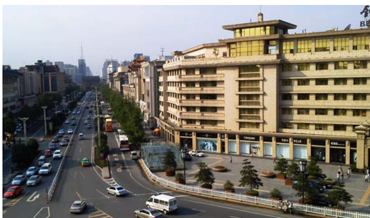
Bell Tower Hotel Xi'an and South Street, as seen from the Bell Tower.
