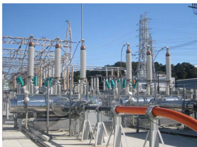
66 kV-class superconducting cable (at Asahi Substation)
