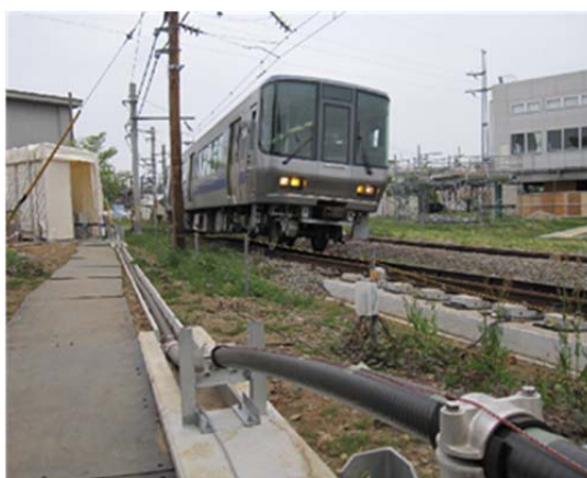
Fig. 1 A 31 m-long superconducting cable installed at a railway line
