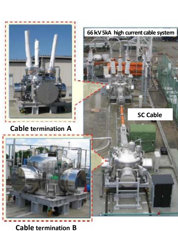
Fig. 3 System outline for demonstration of the 66 kV-5 kA high current cable
