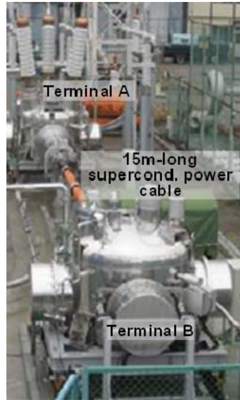
Fig.2 66 kV/5 kA-class large current cable system (Sumitomo Electric Industries, LTD., Kumatori, Japan)
