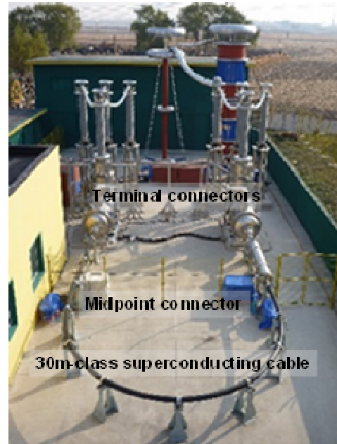
Fig. 6 275kV/3kA-class high voltage cable system (Furukawa Electric Co., Ltd., Jiangsu, China)
